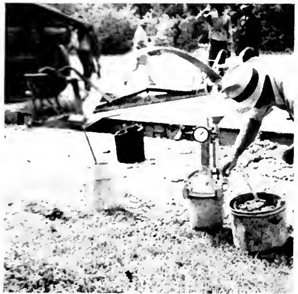
MEASUREMENT IS MADE OF THE AMOUNT OF AIR ENTRAINED IN CONCRETE
